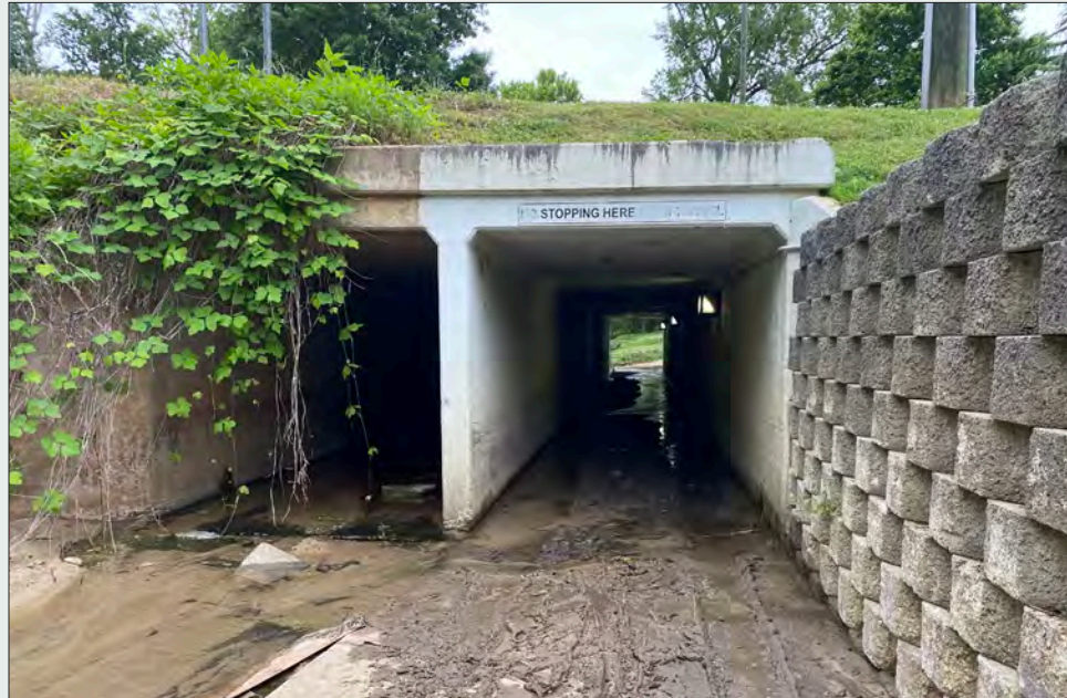
Avon/Catawba Creeks Greenway Underpass
