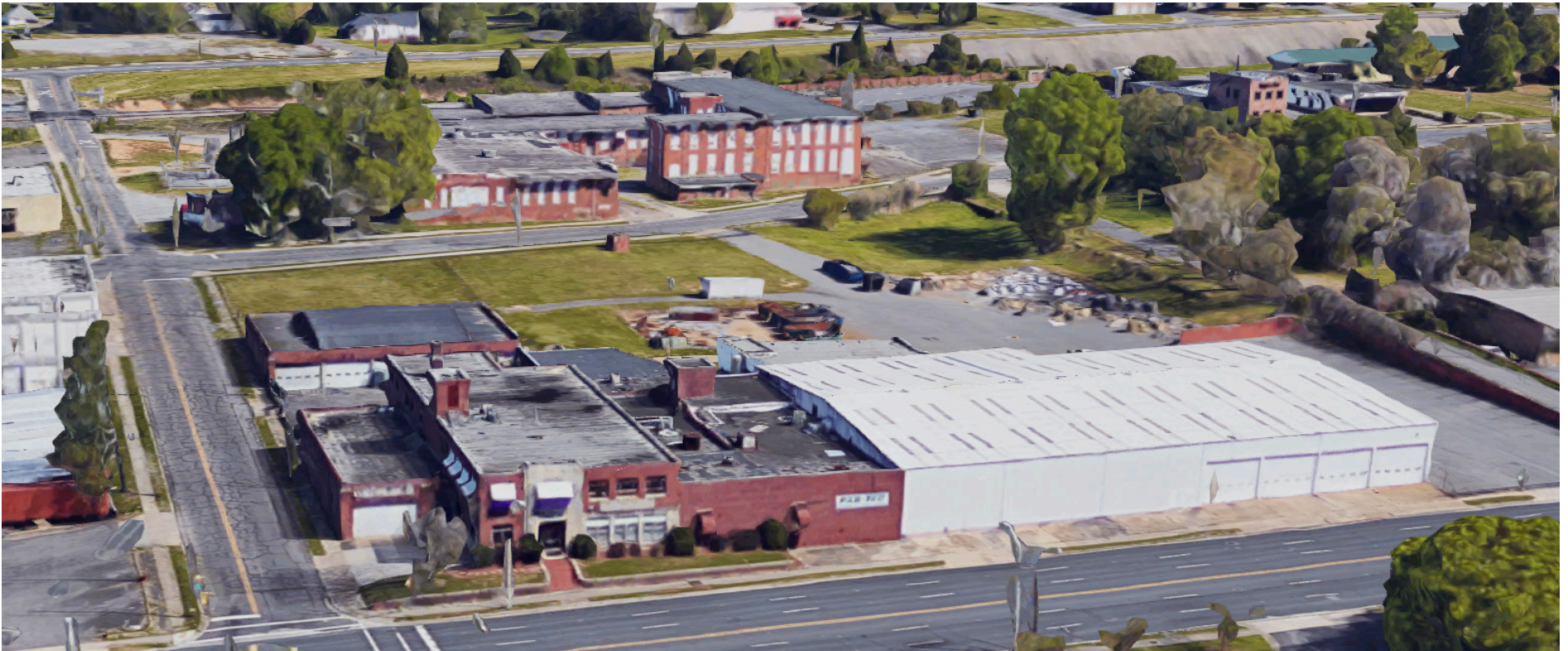
Former Coca Cola Building with Trenton Mill in the background
