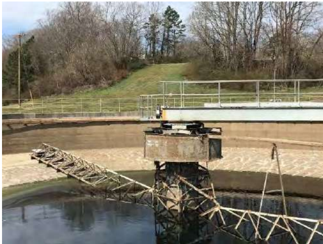
Long Creek Clarifier Rehab
