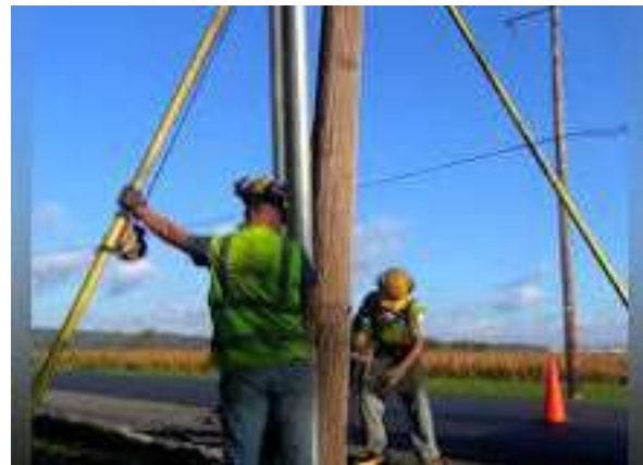
Osmose Pole Inspection
