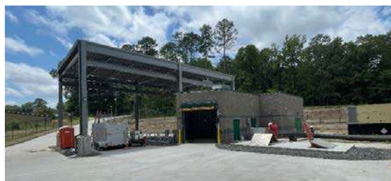
South East Sewer Pump Station Construction
