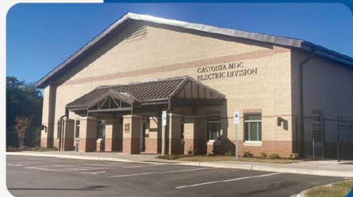
Pictured: Municipal Operations Center - Electric Division
