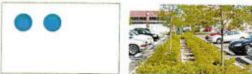
Green Parking Infrastructure: Green infrastructure designed to increase tree canopy for large parking lots and decrease stormwater runoff.
