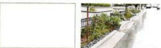
Rain Garden: Vegetated or landscaped depressions designed with an engineered soil layer that promote infiltration of stormwater runoff into the underlying soil.
