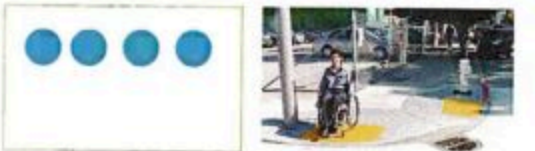
ADA Improvements: Adapt sidewalks to improve mobility for people with disabilities, children and the elderly.
