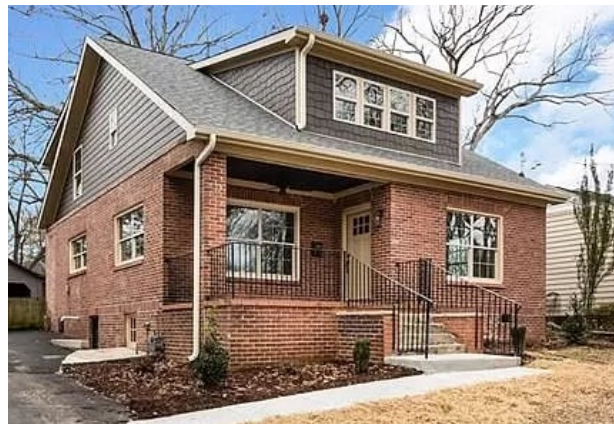
Second floor new construction
