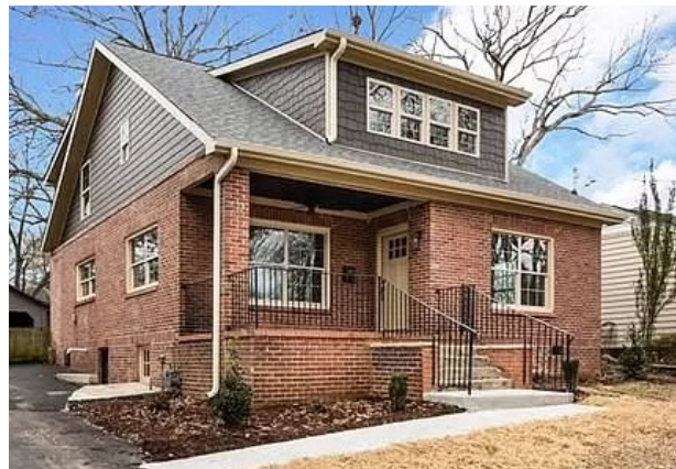
Second floor new construction
