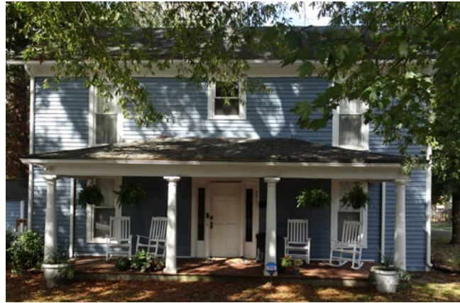
Preserve historic front porch
