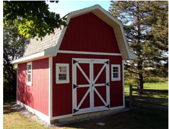
Inappropriate barn-style shed
