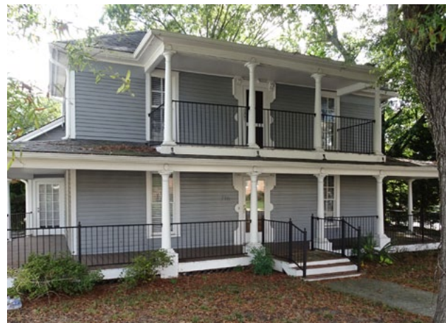
Original decorative door frame features
