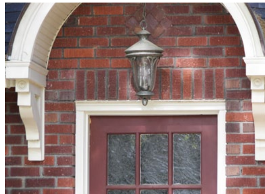
Decorative lighting fixture above front door
