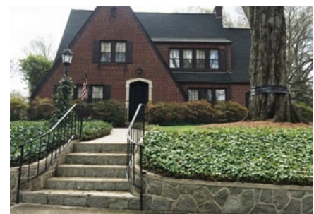
Stone masonry steps & wall
