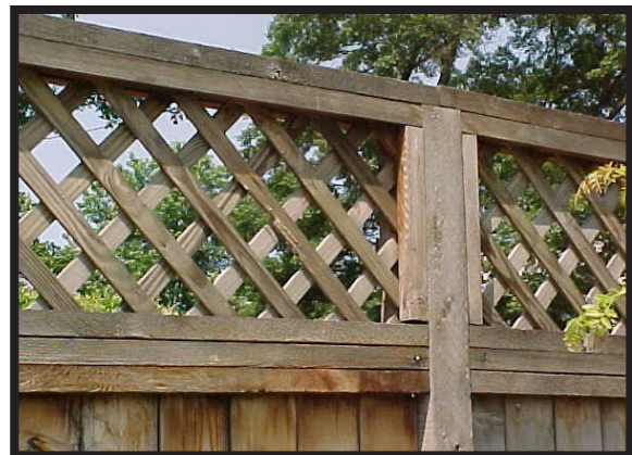
Wood Privacy Fence
