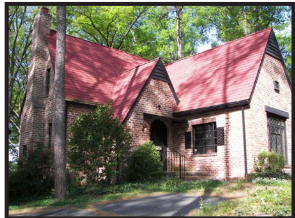
Retain Roof Shape
