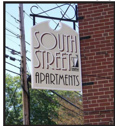
Sign attached to Historic Structure using ornamental metal hardware
