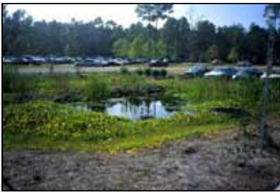
On-site management of stormwater: detention ponds detain stormwater for a period of time and releases it slowly to the drainage system.
