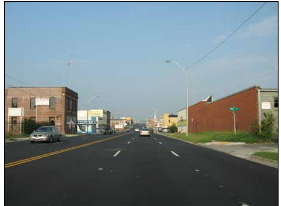
Franklin Boulevard 6 lane configuration
